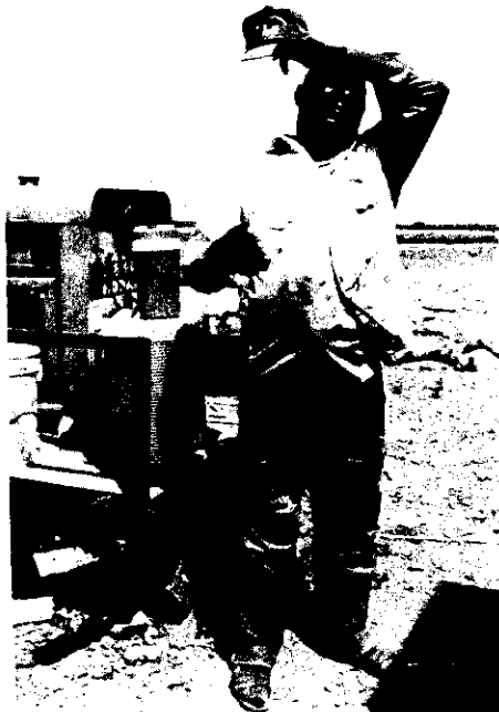
During heat spells, special measures should be taken, such as postponing non-essential tasks and monitoring workers closely for heat stress.
