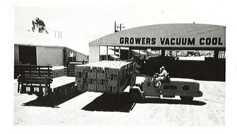
Now a vacuum cooling process chills the lettuce for shipment. Material handling equipment replacing dozens of laborers load the lettuce onto trains or trucks. Within hours the lettuce will be the substance of hundreds of thousands of salads. A lettuce green prospect for consumers but a grim outlook for lettuce workers. A tenth as many jobs as formerly with the standard rate for highly seasonal work less than 90 cents an hour.
