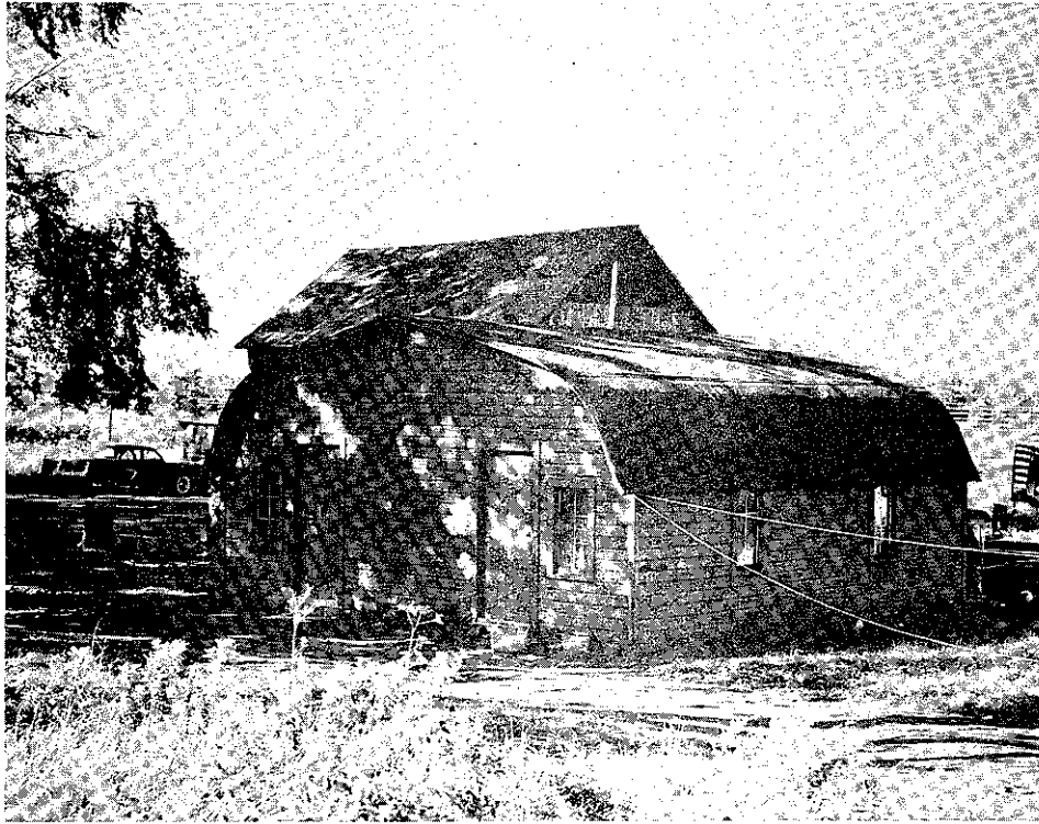
Four-family barracks at Ernest Camp, Whitestown, Oneida County
