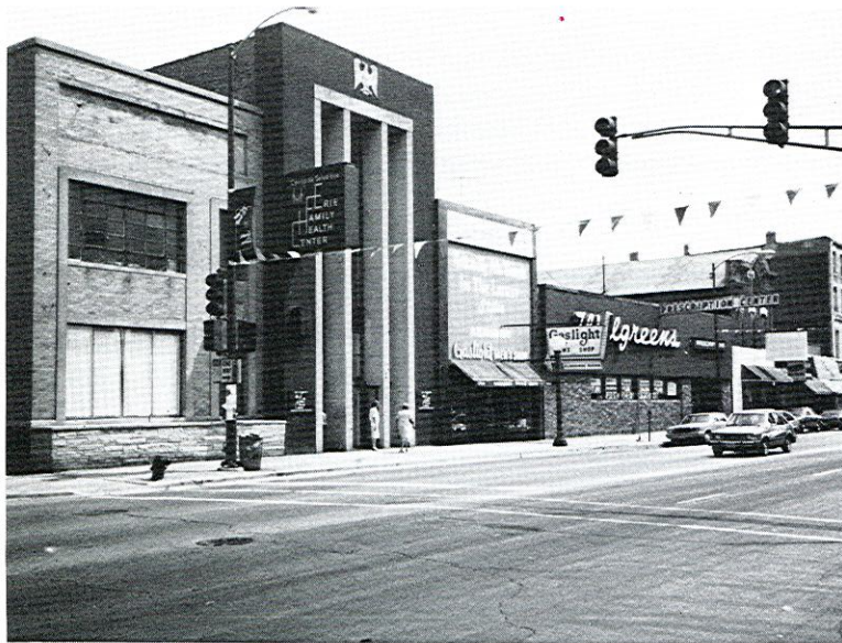
ERIE FAMILY HEALTH CENTER Chicago —The Erie Family Health Center has grown, in the past two years, from a small clinic located in a Chicago settlement house to two handsome, well equipped health centers. The Chicago Avenue clinic (shown) opened in the spring, and the Humboldt clinic will open in late
