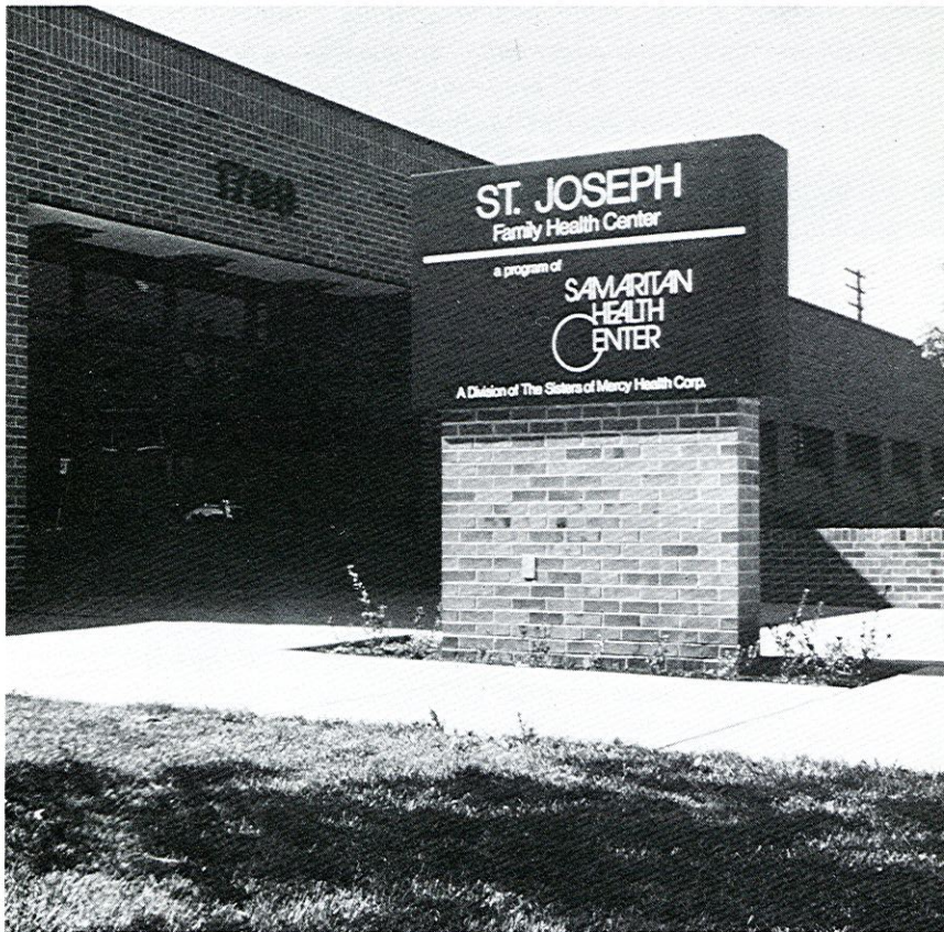
ST. JOSEPH FAMILY HEALTH CENTER Detroit— St. Joseph Family Health Center in Detroit is one of five health centers renovated by the Sisters of Mercy Health Corporation in 1985-86, and the Corporation now plans to establish a new center. By expanding its facilities and adding nineteen physicians to its staff, Sisters will be able to serve almost 20,000 additional patients.
