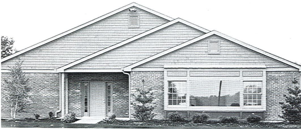
GOSHEN MEDICAL CENTER Goshen, Ohio—With the addition of the Goshen Medical Center (shown) last year and the Batavia Center this year, the Southern Ohio Health Services Network now has eleven health centers serving over 20,000 patients in southeastern Ohio. To further expand its services, the network is planning to provide prepaid care for Medicaid, Medicare, and private patients.
