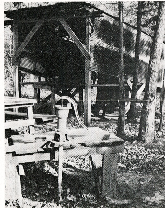
Water supply and cooking facilities at a migrant camp site. To conform with the new regulations, water supply must be protected, pitcher pumps replaced with approved type. Public food preparation areas should be screened against flies.
